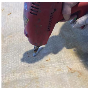
4 | Fill the hole with the polyamide repair filler.
