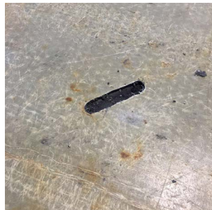
3 | Remove dust using an air compressor.
